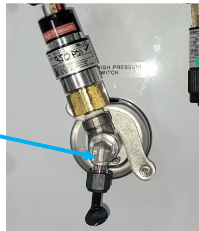
Connect Membrane Pressure Gauge
